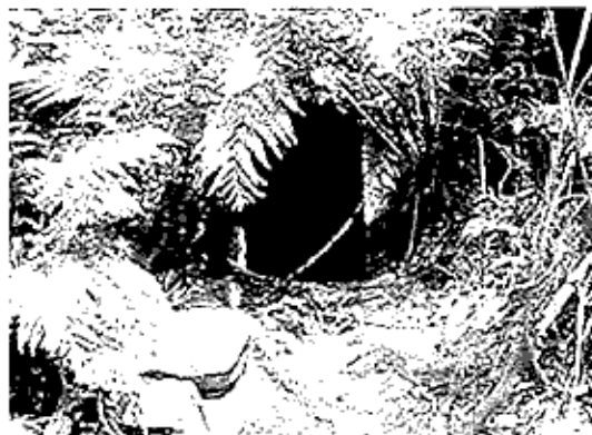
TUNNEL UNDER ST JOHN'S ROAD - built during the war to enable the road to be blown up with explosives if the Japanese invaded. The work of the army in repairing roads etc in the Crater may have been quite extensive. The bridge at the Devil's Elbow was blown up by the soldiers.
