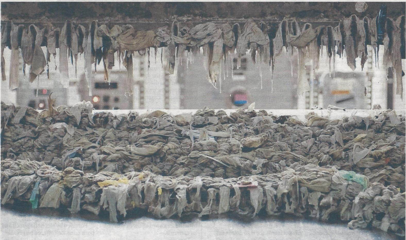
A mechanical rake collects wet wipes that have gone through the plumbing network at a New York water treatment plant. Photo: New York Times
